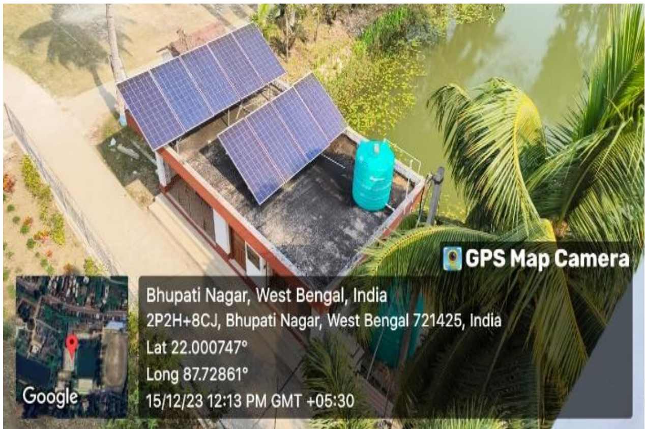
Solar Panel installed on the roof of the pond water purifier house
